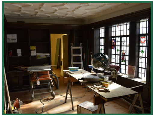
Construction within 605 Fillmore
